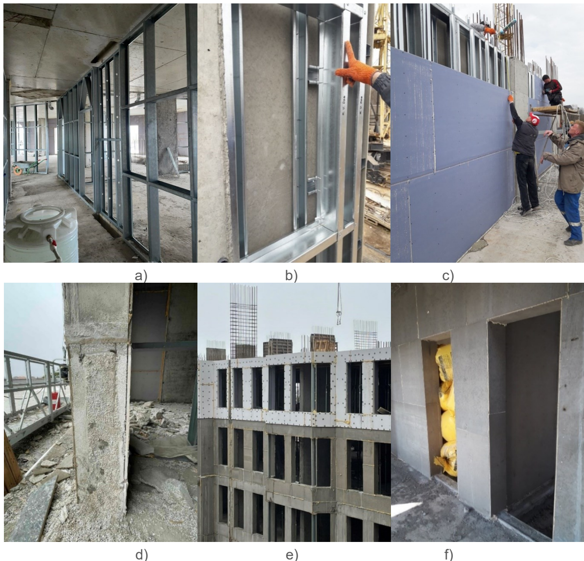
Figure 11. Process of erecting the developed solution of the enclosing frame structure using expanded polystyrene concrete in a fixed formwork: a) erecting the frame from LSTWS; b) assembly nodes of the frame from LSTWS; c) sheathing the frame with cement chipboards; d) concreted wall; e) external view of the finished structure from the outside of the building; f) external view of the finished structure inside the building
