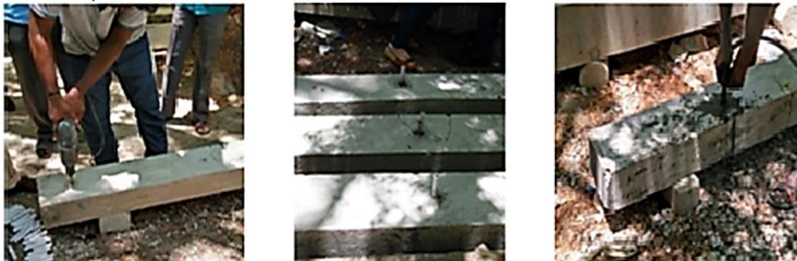
Figure 3. Grouting process for the pre-damaged beams
