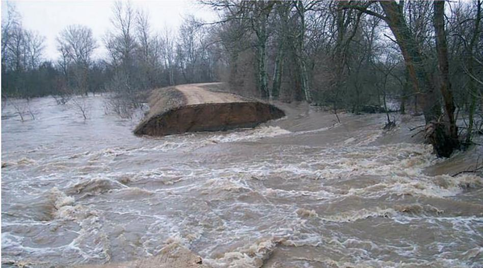
**Figure 9.** Levee break in the flood of 2006 (Malkarali et al., 2008).
