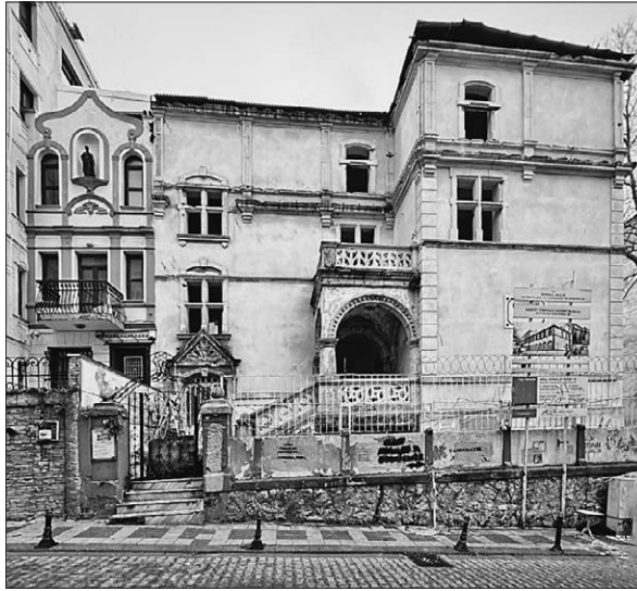
FIG. 3 SCHOOL'S NORTH FACADE FROM İSKELE STREET
