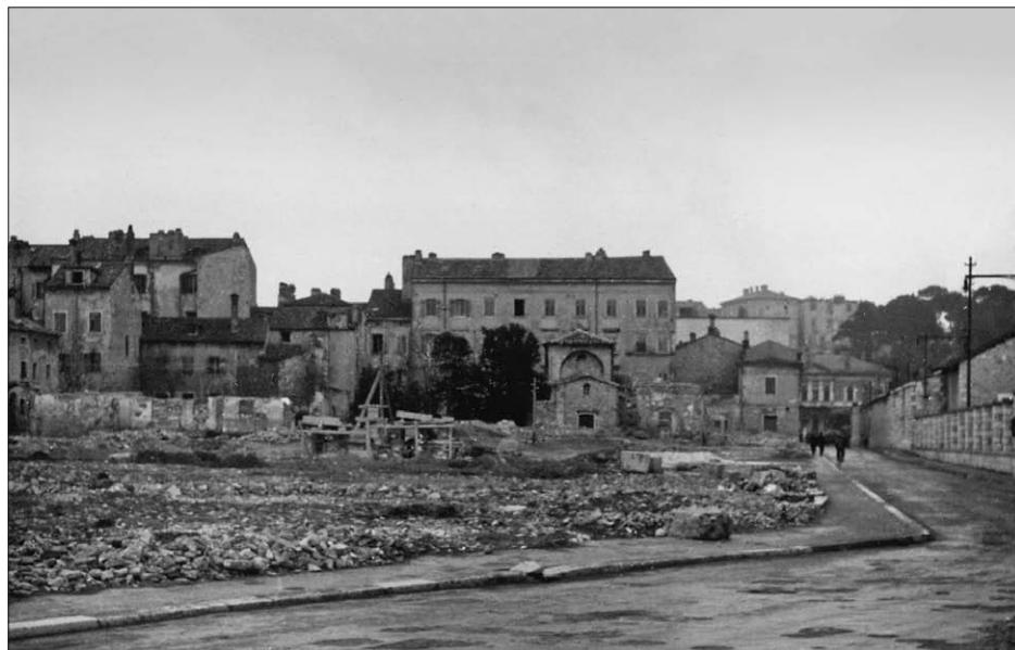
FIG. 10 BLOCKS 21 AND 22 AFTER DEMOLITION IN 1953
