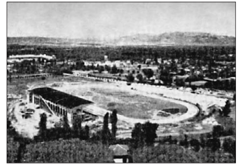
FIG. 9 VIEW OF THE BURSA STADIUM IN 1948
