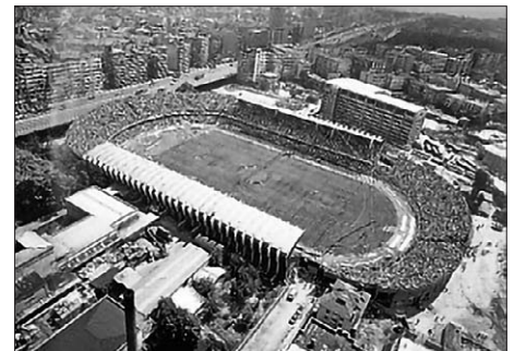
FIG. 11 AERIAL VIEW OF THE GALATASARAY STADIUM
