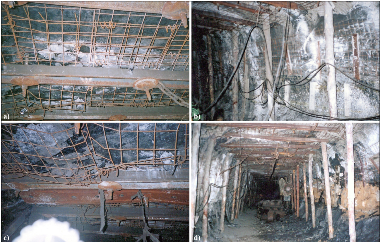
Figure 11. Condition of the rocks of the roof (a, c) and sides (b, d) of the conveyor roadway of the northern main longwall of seam k_8^u at a distance of 25-30 m before the face (a, b) and 25 m after the face (c, d)
