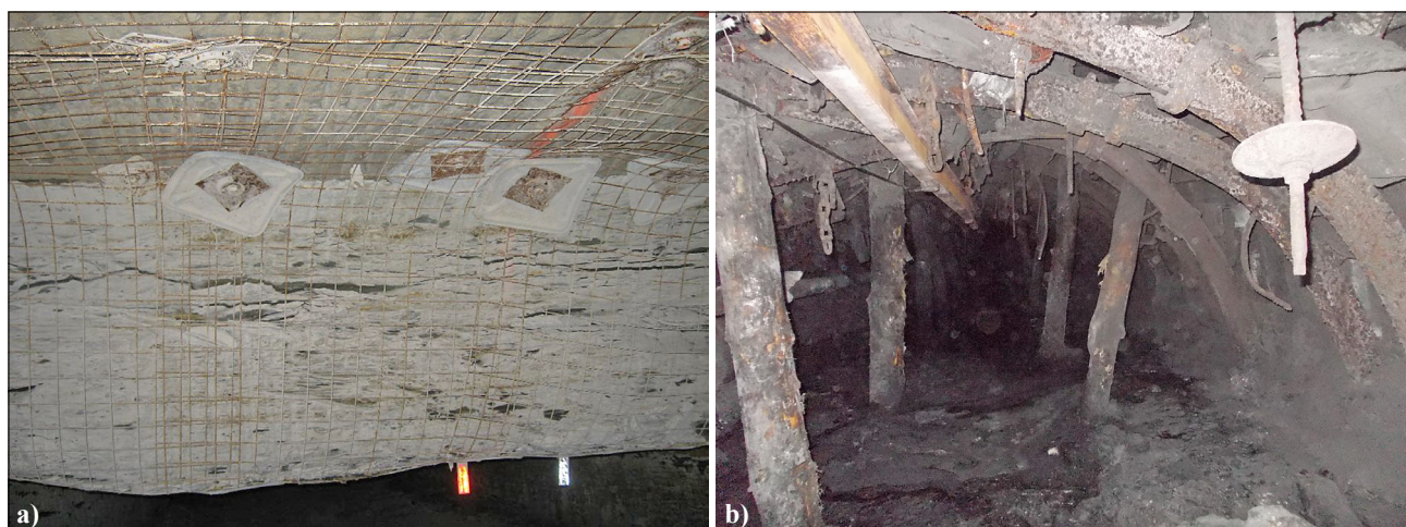
Figure 12. Bed separation in weak shale fixed by rock bolts a) Collections Illinois, USA (Molinda and Mark, 2010) (b) Management Board of the «Pokrowskoje» Mine, Ukraine (authors' photo)
