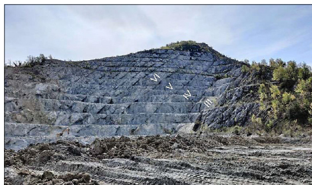
Figure 1. Eastern view of the quarry, with evidenced the four gypsum layers currently under excavation (Marabini & Poli, 2021)
