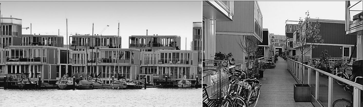
FIG. 2 VIEW OF WATERBUURT-WEST FLOATING NEIGHBORHOOD, IJBURG, AMSTERDAM
