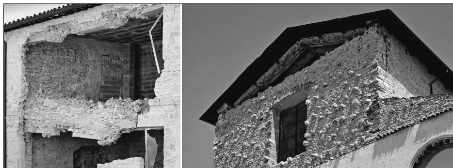
FIG. 2 INADEQUATE STRENGTHENING METHODS (BINDA AND MODENA, 2011)
