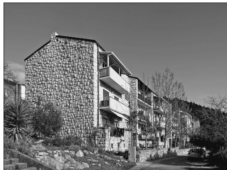
FIG 6B PHOTOGRAPH OF RESIDENTIAL BUILDINGS AT VLADIMIRA NAZORA STREET 13 (ARCH. BRANKO DOŠEN) AND VLADIMIRA NAZORA STREET 15-17, 19-21, 23-25 (UNKNOWN AUTHOR), SOURCE: AUTHORS
